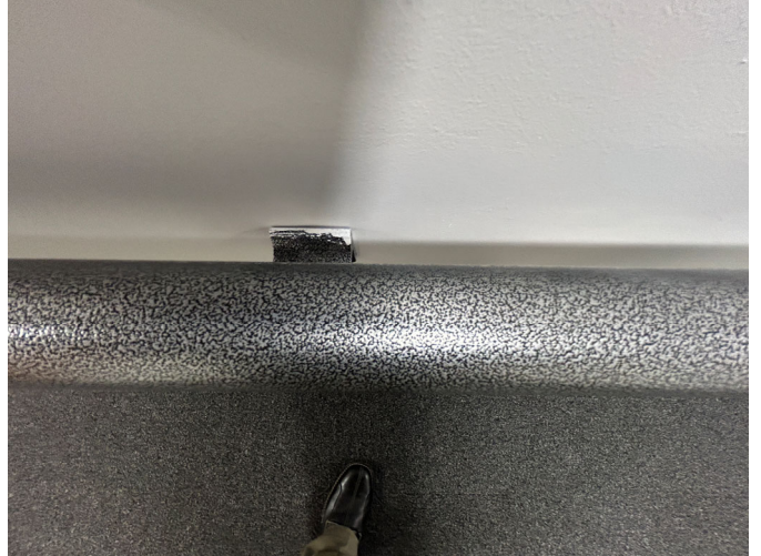
Wall paint visible on handrail brackets in corridor.
